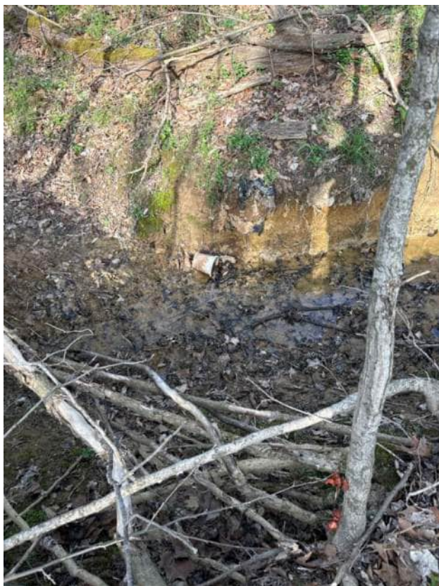
ID: S-BS-5-3 Date: 4/14/2026 Direction: N Position: Across
